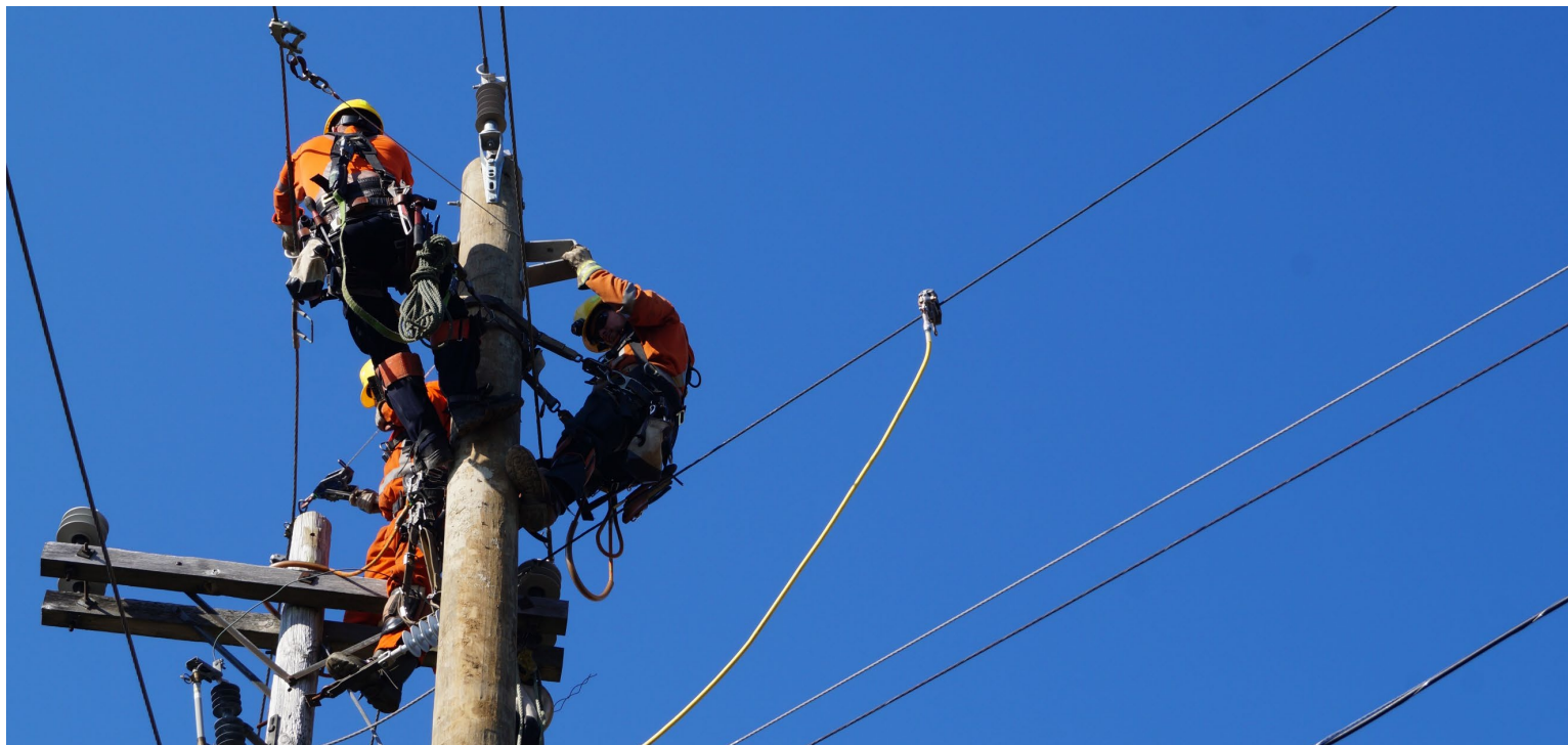
Photo: Crews replacing a crossarm structure.
